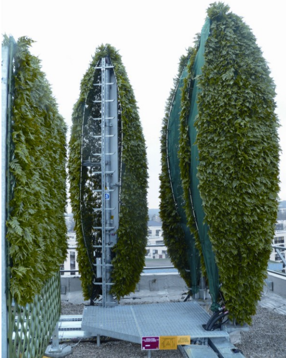
Example of landscape integration of antennas on a town hall roof in the municipality of Le Chesnay (Yvelines, France).
